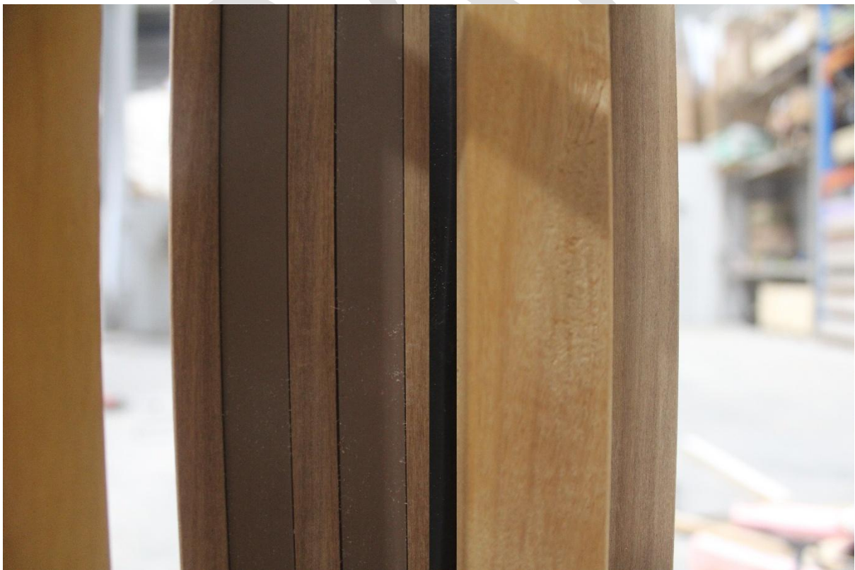
Figure 19 – Frame seals, smoke seal and door stop on door frame
